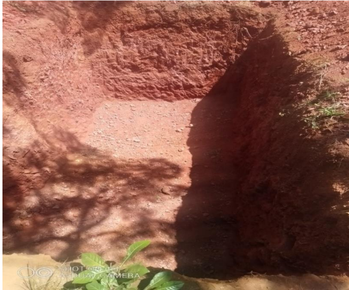
The septic tank awaiting construction
